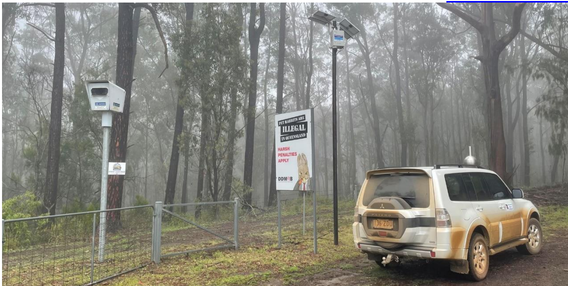
Ongoing surveillance, repair and replacement maintain the effectiveness of the Darling Downs-Moreton Rabbit Fence.
